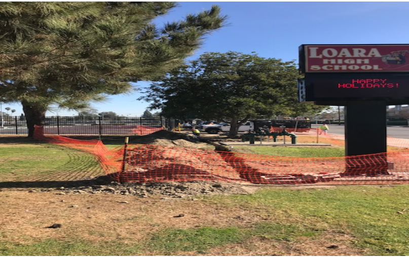
Conduit for motorized gate @ Teacher's Parking
