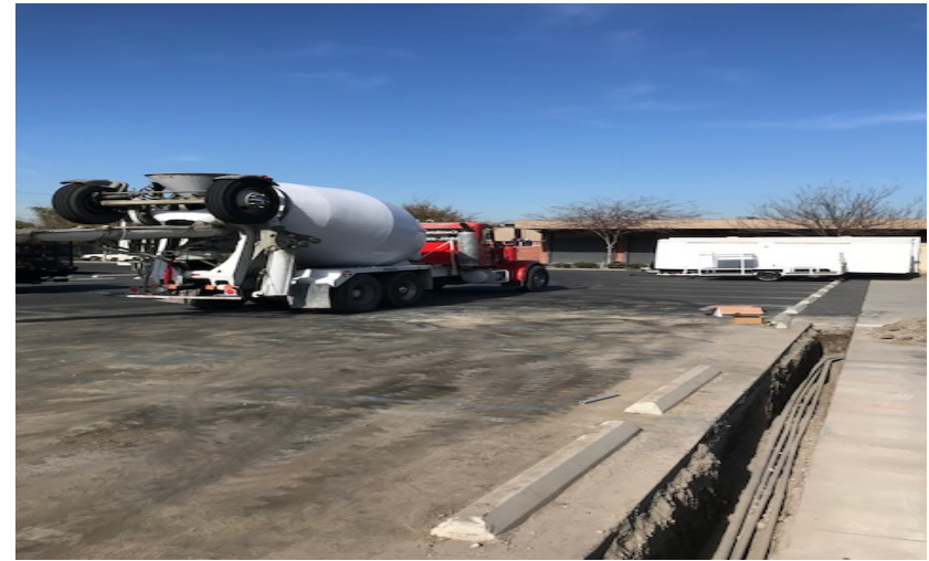
Trench for motorized gate conduits @ West Service Rd.
