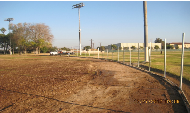
Contractor installing fence posts at City Baseball Field
