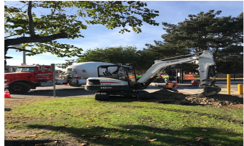
Trenching/Concrete temp. patch
