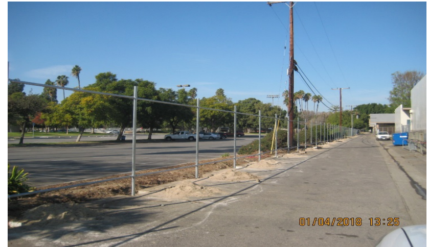
Contractor installing fence posts by Alley
