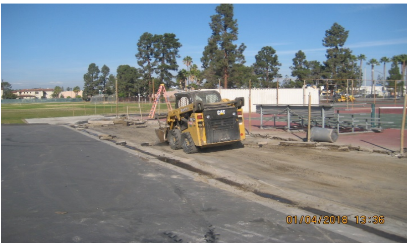
Contractor installing fence posts at Tennis Courts
