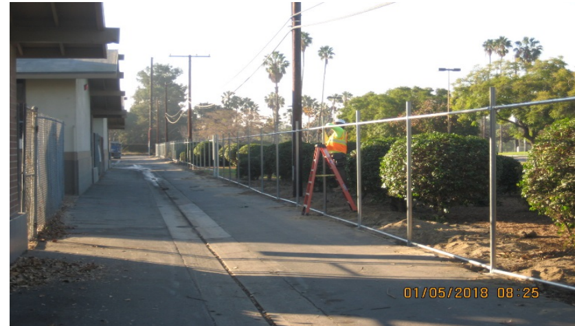
Contractor installing fence posts by Alley
