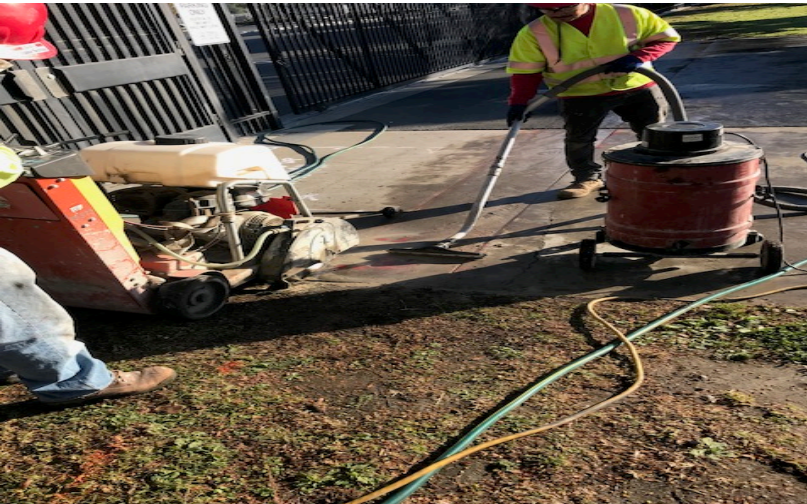
Temp. patch of trench for gate operator
