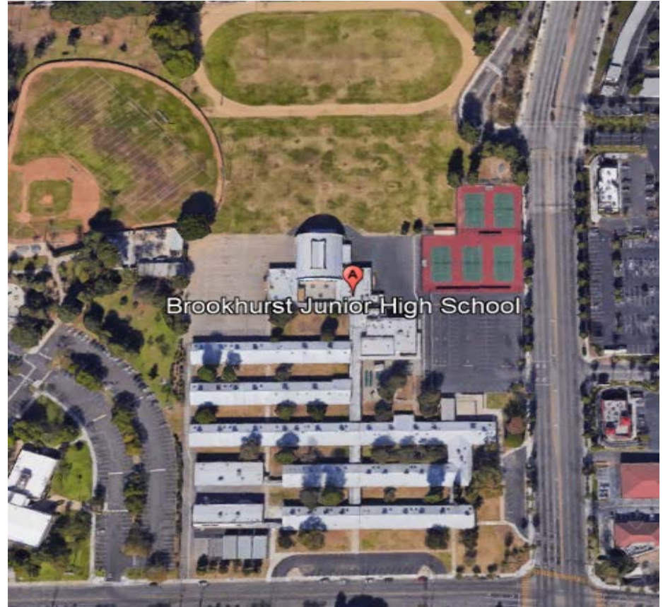
Measure H funding will be used to fund security fencing.
